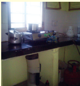
The dysfunctional water purifier in MTC Gola (Ramgarh)
