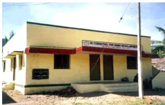
Schools having inadequate capacity
